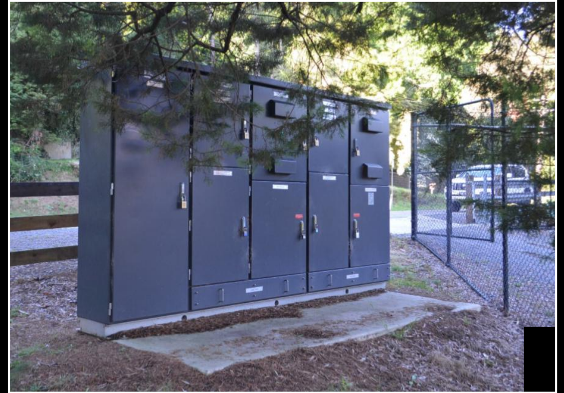
TYPICAL SEWAGE PUMP STATION MAIN SWITCHBOARD
